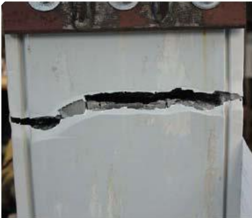
(a) Failure @ 0.003 in/sec Stroke Rate
